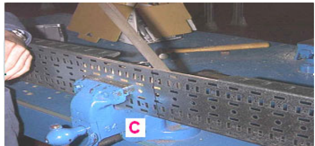
Figure 85: Construct a flat Bend 90° (C)
